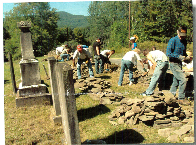
Elkdale Cemetery Stone Wall Repair Project
